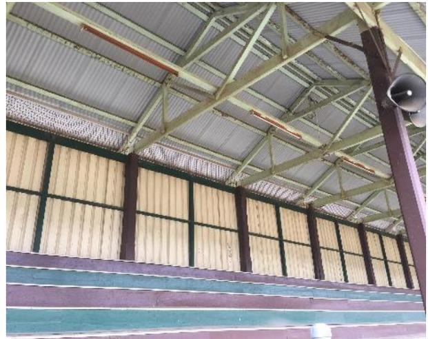
Figure 8 roof trusses and seating in the old grandstand
