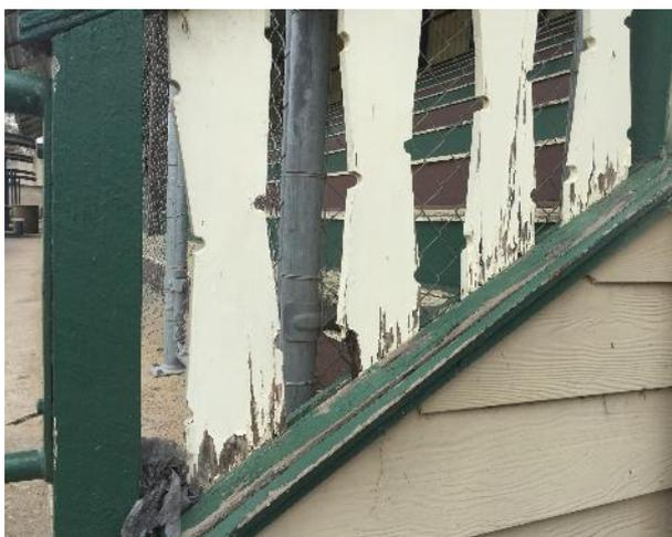
Figure 9 Damaged timbers on the northern facade
